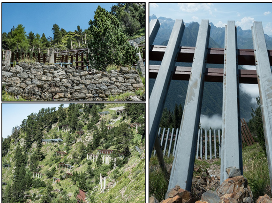
Figure 6 Anti-avalanche defences in the Thiel corridor
