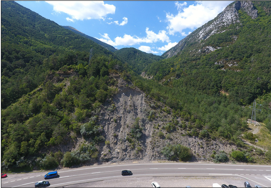
Figure 19 Front view of the Santa Elena roadcut.
