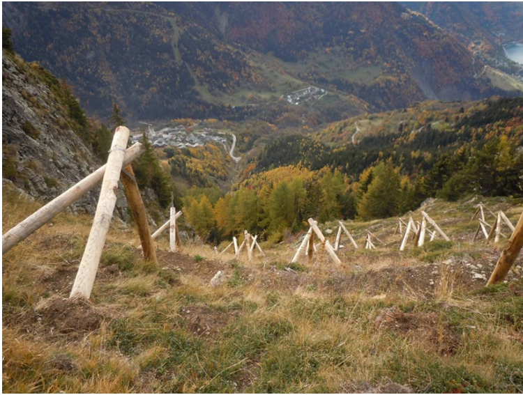
Figure 70. The type of wooden structures, made from local wood, planned for implementation to protect the plants from damage by snow creep during the first years. The structures will themselves also prevent release of snow avalanches (Solheim et al. 2019)a
